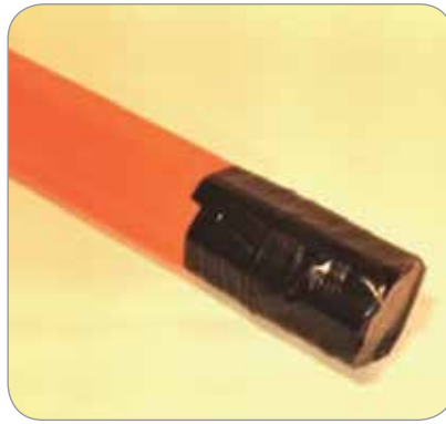
Sealing the End of FuturePath Prior to Installing a Pulling Grip
