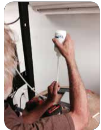
Bend the duct into a gentle U-shape with the tail at the desired length required for the fill.
